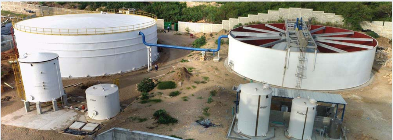
Complete Water treatment system with 3000USgpm (680m 3 /hr) Solid contact clarifier, chemical injection units (3), 4000m 3 storage tank, residuals thickener unit.
